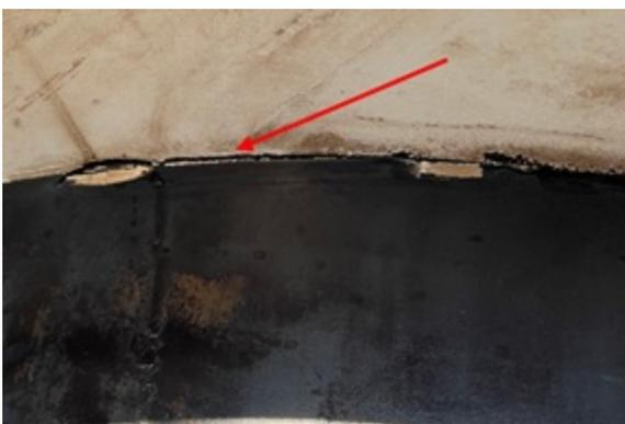
*Figure 2: Insulation at blind flange.*
