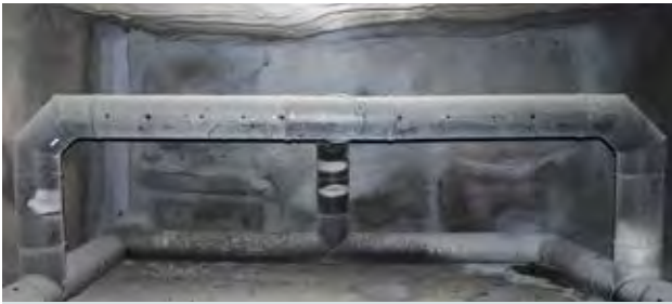
A series of 14-in. HDPE drainpipes is placed in each plug to direct water down the mountain.
