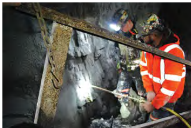
Miners pump AFS into the rib to seal against water ingress.
