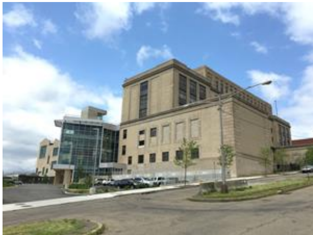
(2) Capstone C65 Microturbines provide Combined Cooling, Heating & Power (CCHP) to the Energy Innovation Center in Pittsburgh, Pennsylvania.
